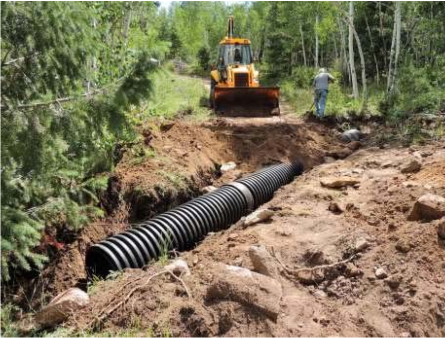
Installation of culvert and access road improvement efforts. August 2017
