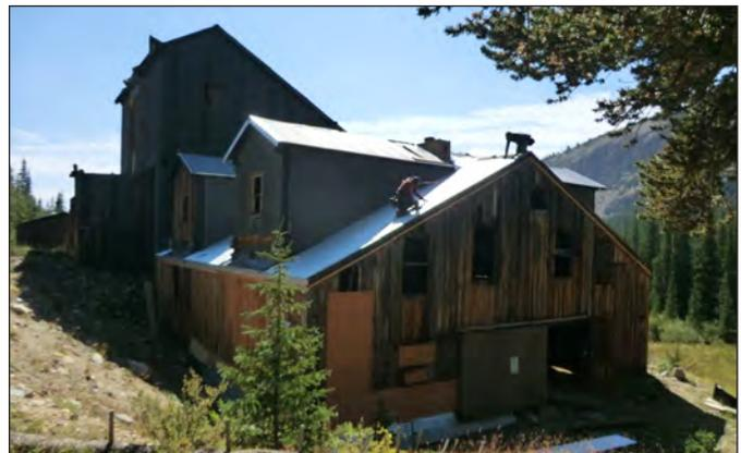
*Workers are putting the final touches on a new roof over the Paris Mill's cyanidation wing.*
