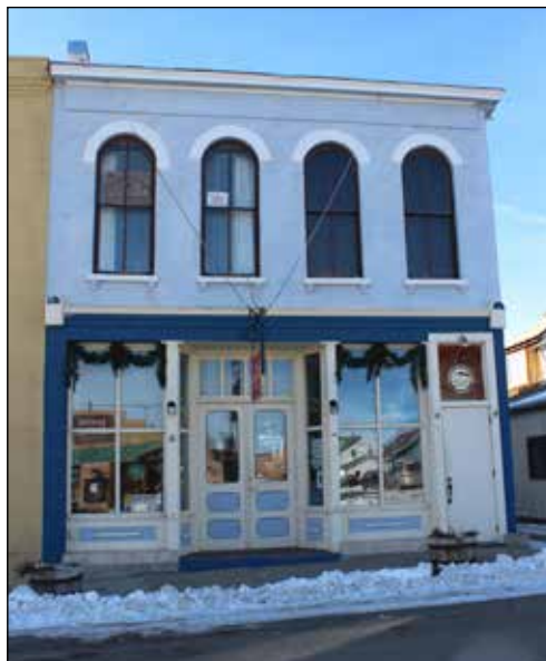
The South Park No. 10 Odd Fellows Lodge was able to repair the roof at its historic hall in Fairplay thanks in part to a PCHPAC grant.
