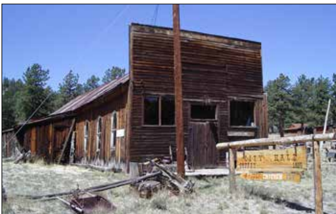
Constructed in 1896, the historic Guffey Town Hall hosted town functions and dances. The false front building now serves as an informal museum and community gathering space.
